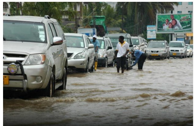
Blocked drainage system at Shoppers Plaza
